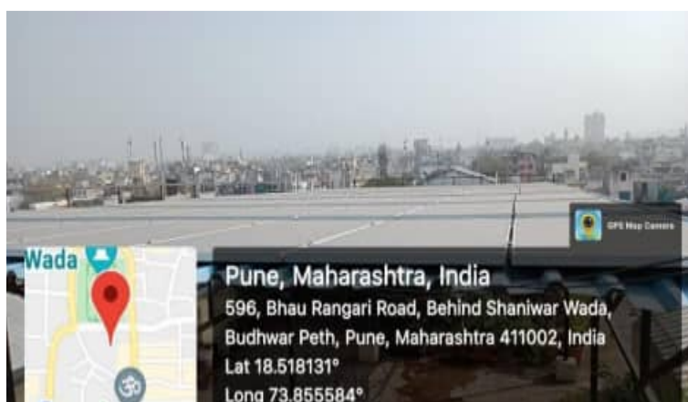
Photograph of Roof Top Solar PV Plant:
